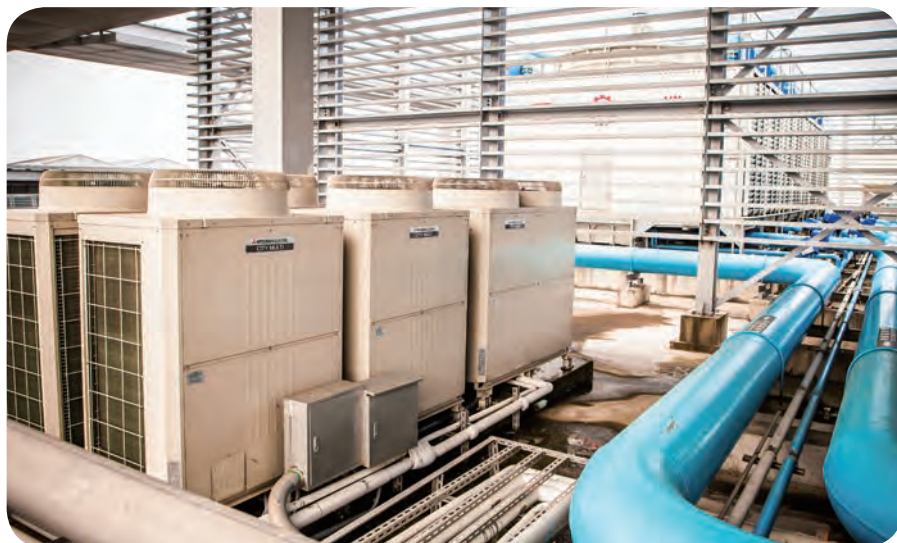
Installation of independent AC
